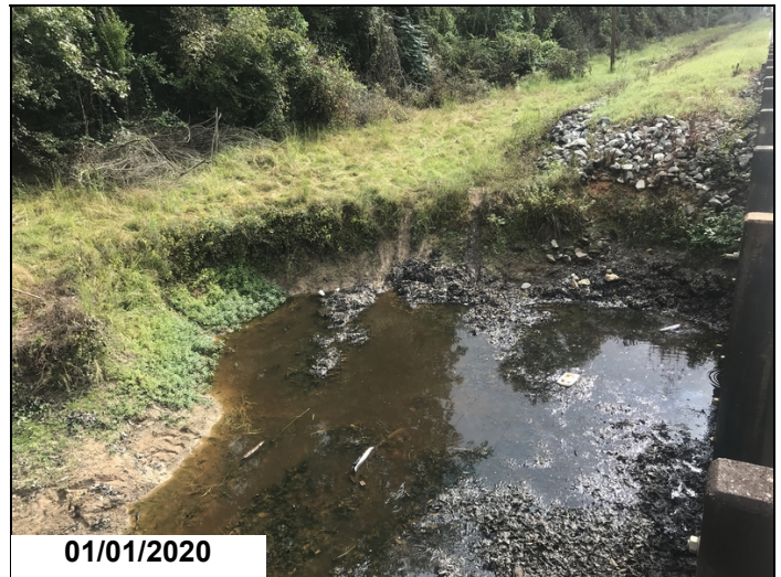
Left side spans 3 and 4, erosion to slope and ditch line.
