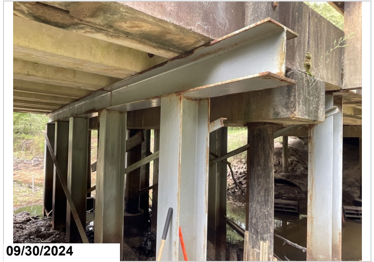
Span 3, supplemental Bent, 2' 3" ahead of Bent 3. Steel columns and steel cap.
