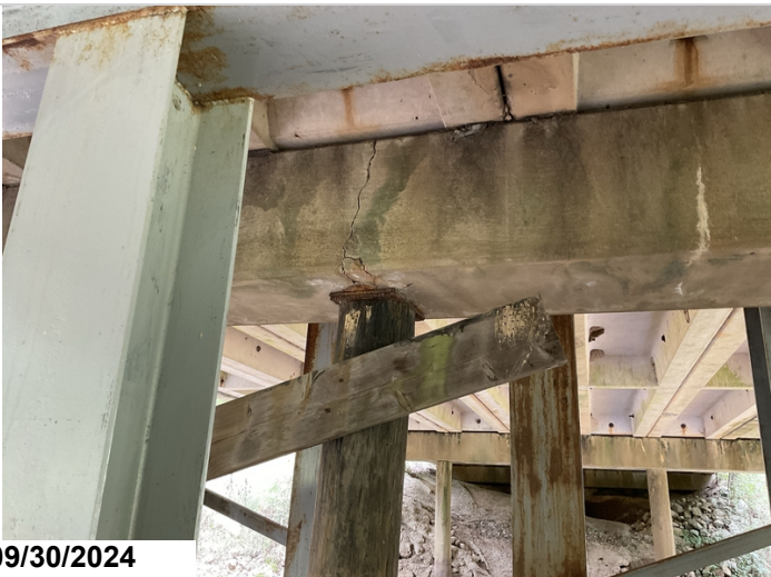
Bent 3 cap cracked over pile 3
