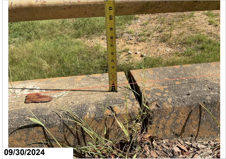
Bent 3 left side, previously cap has dropped causing 1 1/4" sag in curb.
