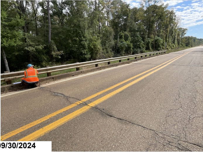
Bent 3 left side, previously cap has dropped causing 1 1/4" sag in curb.
