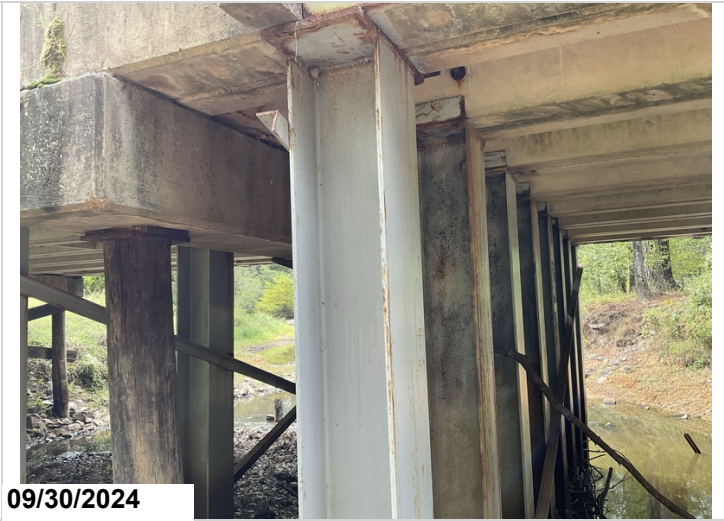
Span 2, supplemental Bent, 2' 0" back of Bent 3. Steel columns with steel saddles under the channel unit legs.
