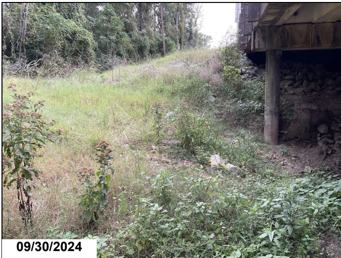
Bent 4 and 5, scour repairs have been made.
