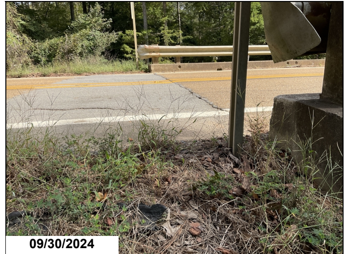
Bent 1 end, road way is settling due to erosion of embankment below the abutment stub.
