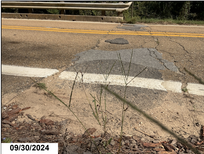
Bent 5 end, road way is settling due to erosion of embankment below the abutment stub.
